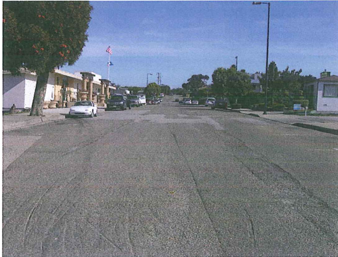
Figure 2: Market Ave looking North
